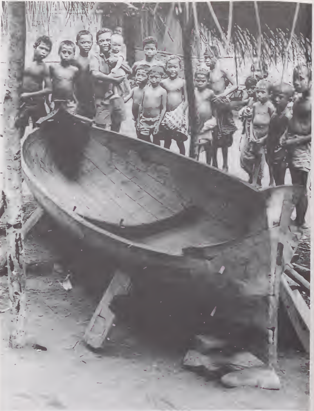
Fig. 6. The plank shell of a sapa nearly complete; the planks have been reduced in thickness and smoothed.
